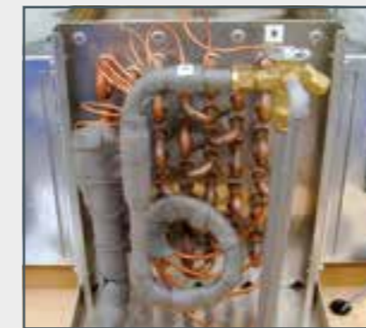
Direct evaporator as air cooler
