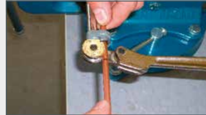
Inserting the pipe into the bending device
