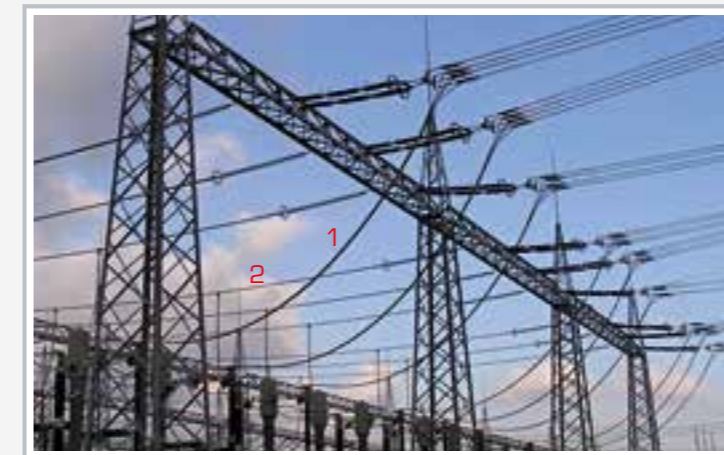
Free-hanging cables in practice (portal): 1 stay cable, 2 power line, similar to overhead line
